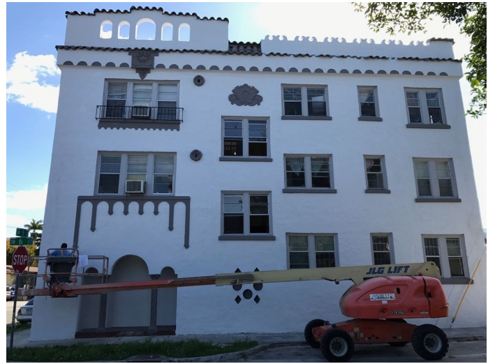
NEW ROOF COMPLETED!
